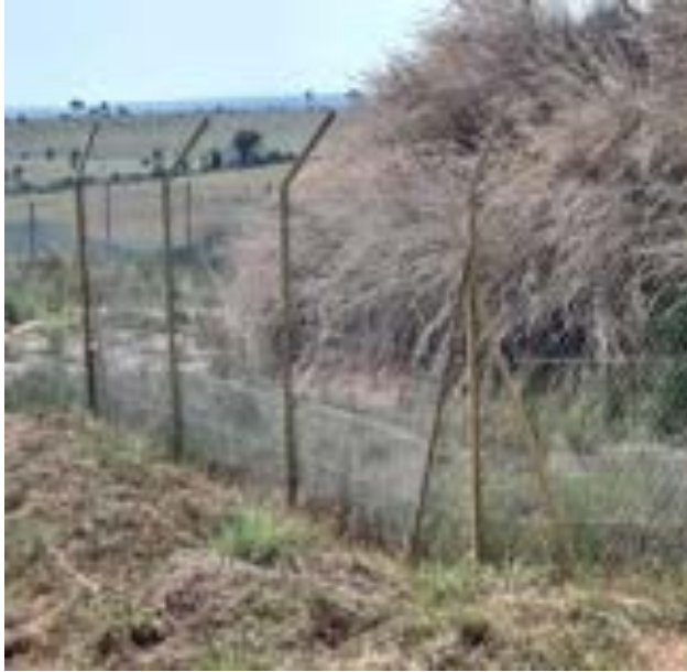
Vegetated bunds around well pads. The exterior fence will be removed.
